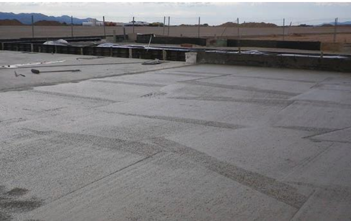
Plaveisel vliegveld – Aeródromo T-35, AVIALSA, Spain. 5 kg/m 3 Anti-CRAK® HP 67/36, C 30/37.
